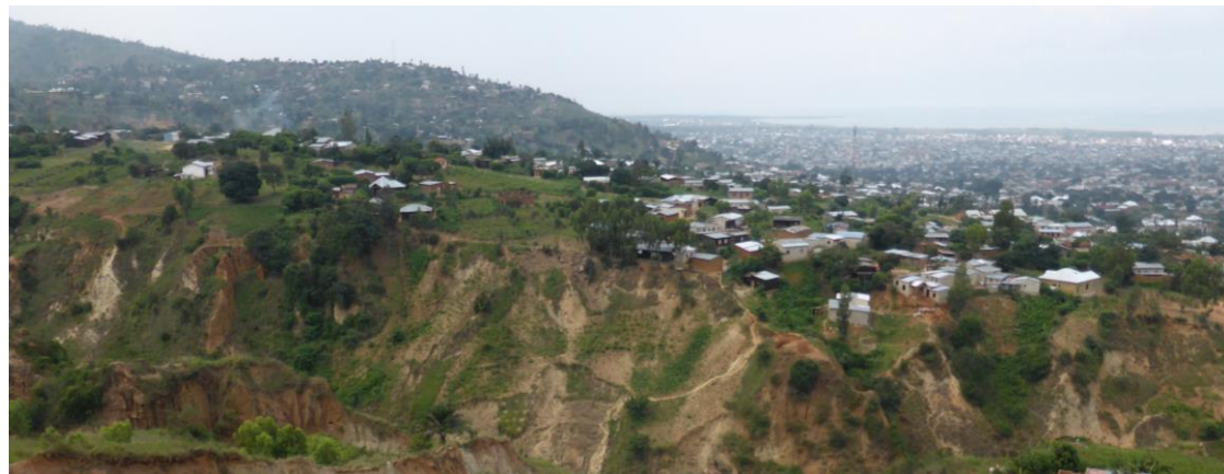
Large (urban) gullies – landslides
